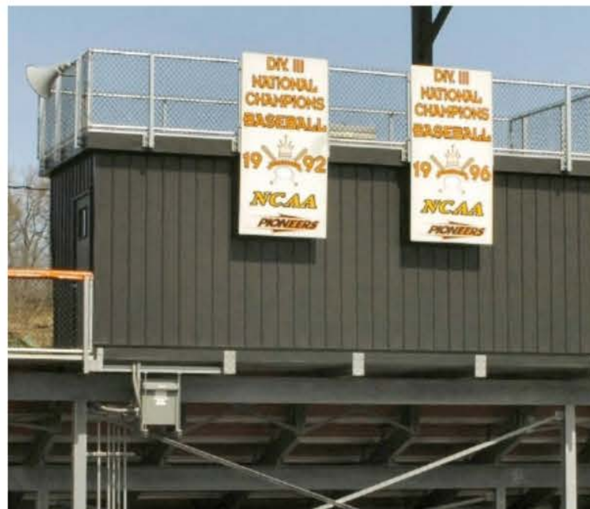
Stadium Press Box
