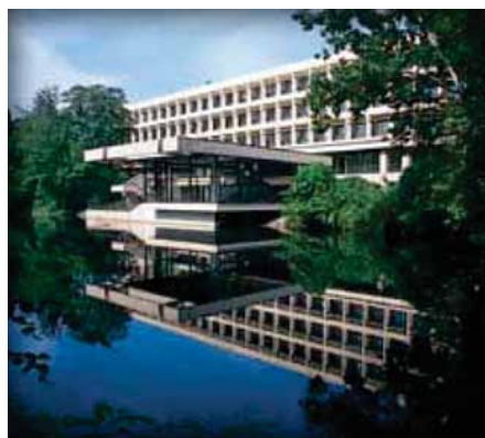
THE BUILDING AT 1600 VALLEY ROAD, WHICH PRESIDENT SPEERT CALLS PIVOTAL TO THE UNIVERSITY'S RECENT GROWTH
