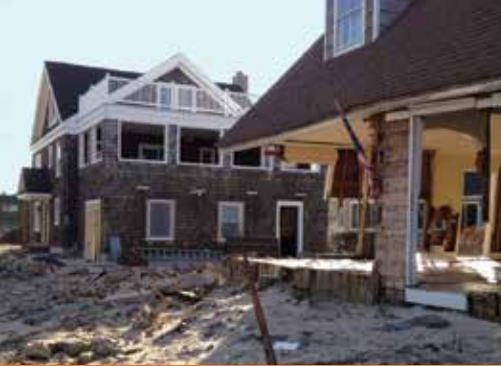
HARD-HIT BEACHFRONT HOMES IN MANTOLOKING
