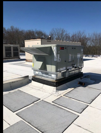
New Energy-Efficient RTU's
