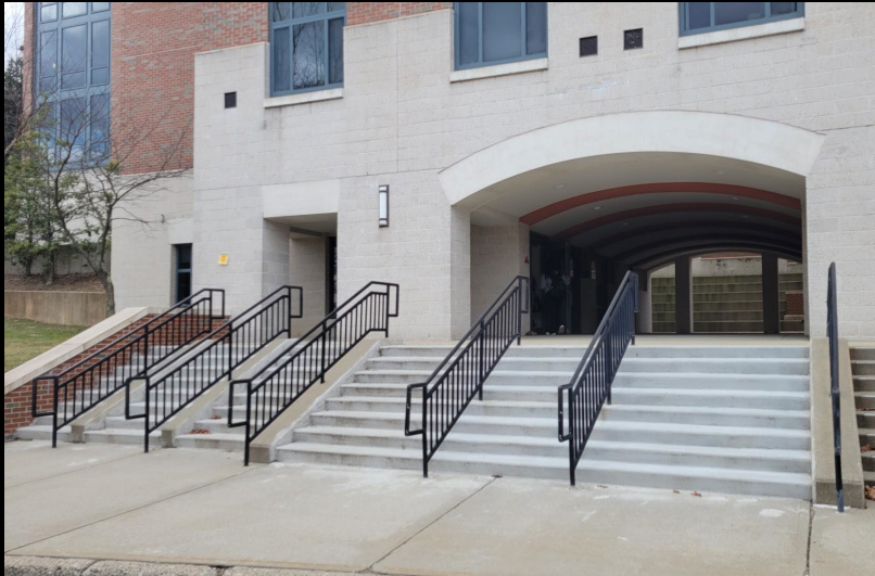
Restored Concrete Entry Steps
