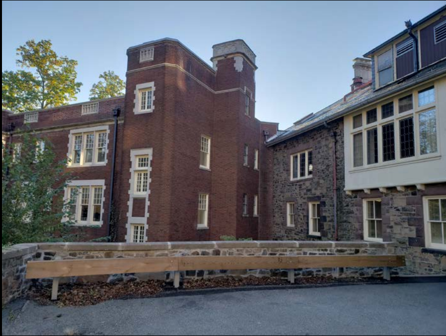
New Guardrail & Restored Retaining Wall
