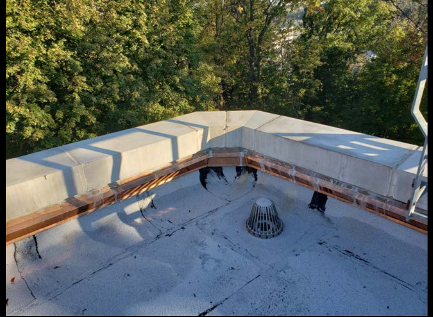
Coping Stone & Flashing Detail
