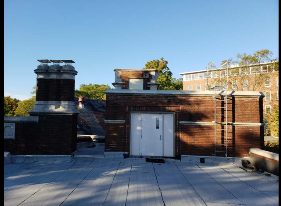
Elevator Penthouse Coping & Roof Replacement
