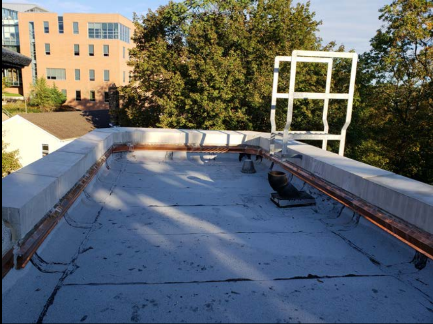
New Flashing, Roof & Cast Stone Coping
