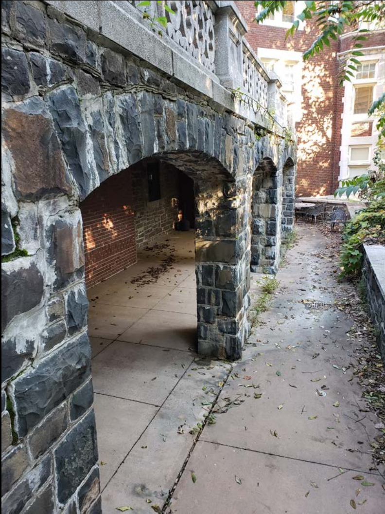
Lower Level Archway Restoration
