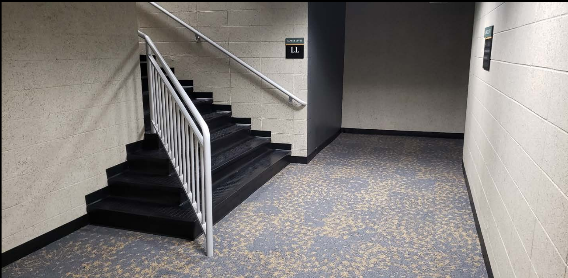
Lower Level Stairs and Landing
