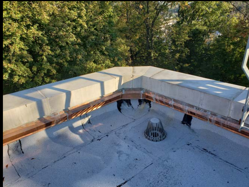
Coping Stone & Flashing Detail
