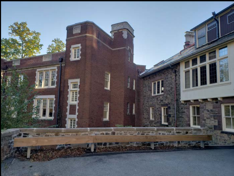
New Guardrail & Restored Retaining Wall
