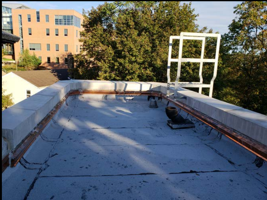
New Flashing, Roof & Cast Stone Coping
