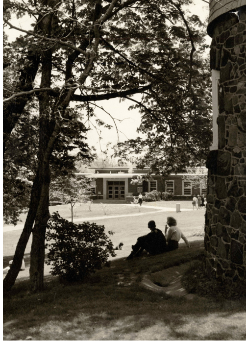
Graphic 3.4 Pump House in Early 1960s (before construction of Raubinger Hall)
