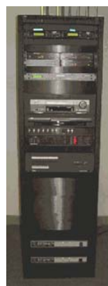
Equipment Tower , located in the room's AV closet
